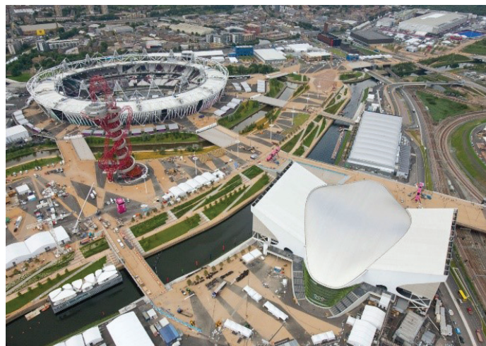
Figure 2: Completed Aquatics Centre during the Olympic Games (picture by LOCOG)
