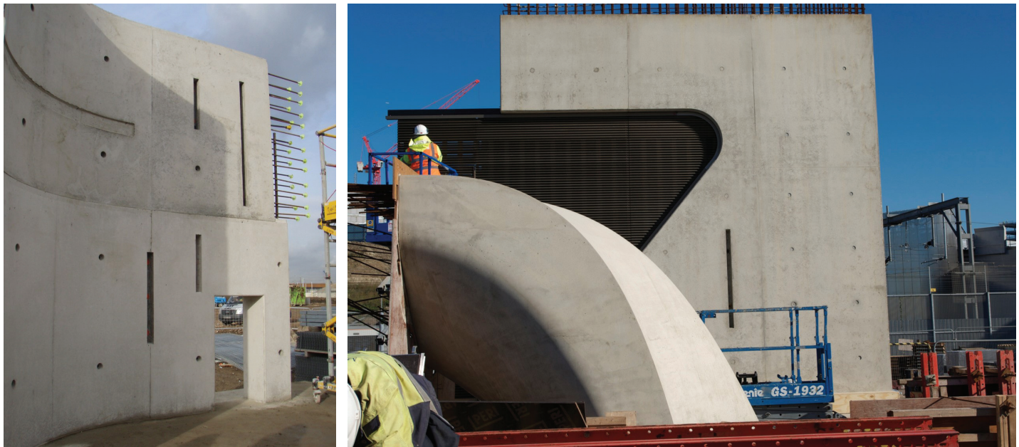
Figure 6: Concrete trial pours and quality control mock ups
