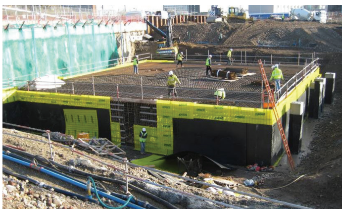
Figure 5: Transfer Structure - largest pour in the Olympic Park: 1800 m 3
