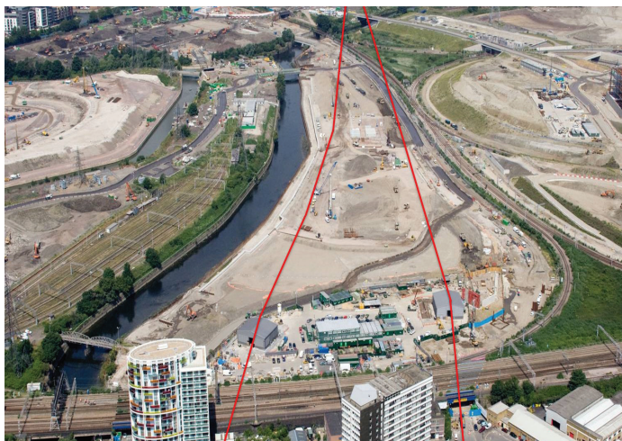
Figure 1: Aquatics Centre site with the underground power lines (picture by LOCOG)
